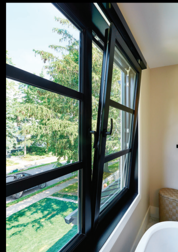
Tilt function promotes natural ventilation without air flow. The partial opening at the top of the sash limits the risks of break-ins, plus protects from injuries or accidents.
