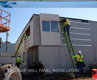
Corona del Rey Affordable Housing Units Corona, California Dryvit Prefabricated Wall Panels | WTI Installation and Maintenance
