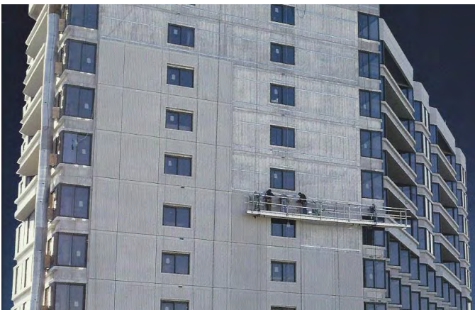
Fedderlite MP restoration over split-faced block
